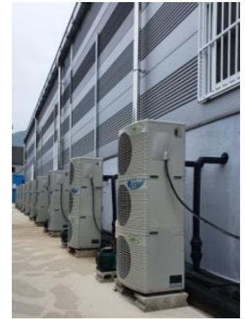
Individual Cooling System of each water tanks
