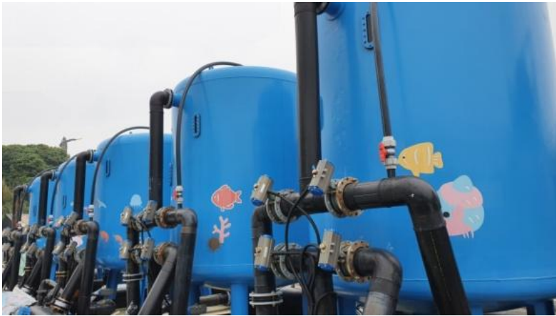
Filtration system for seawater
